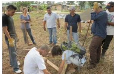
WORKSHOP GROUND RESEARCH AND PREPARATION OF THE FOUNDATION
