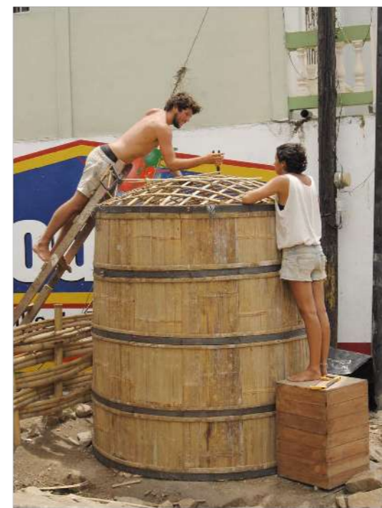
CONSTRUCTION OF BAMBOO WATER TANK
