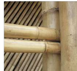
BAMBOO RAIL DETAIL
